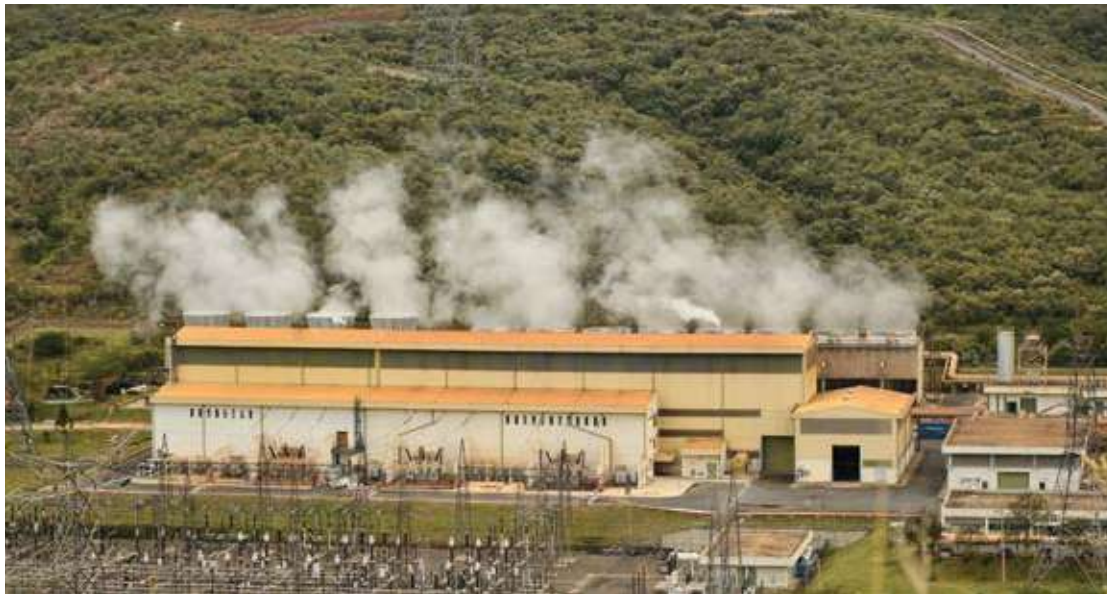
One of the geothermal generating power plant at Olkaria area of Naivasha where Kenya Generating Electricity Company (KenGen) has established an over 8,000-acre green energy park where investors will access direct and lower power tariffs, relaxed customs and tax reliefs. PHOTO: ERASTUS GICHOHI
